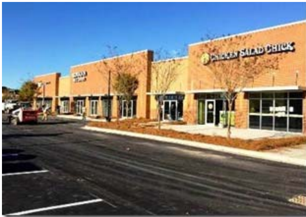
The 11,966-square-foot Shoppes at Azalea building on Azalea Square Boulevard in Summerville was recently sold for $5.2 million. (Photo/Marcus & Millichap)
